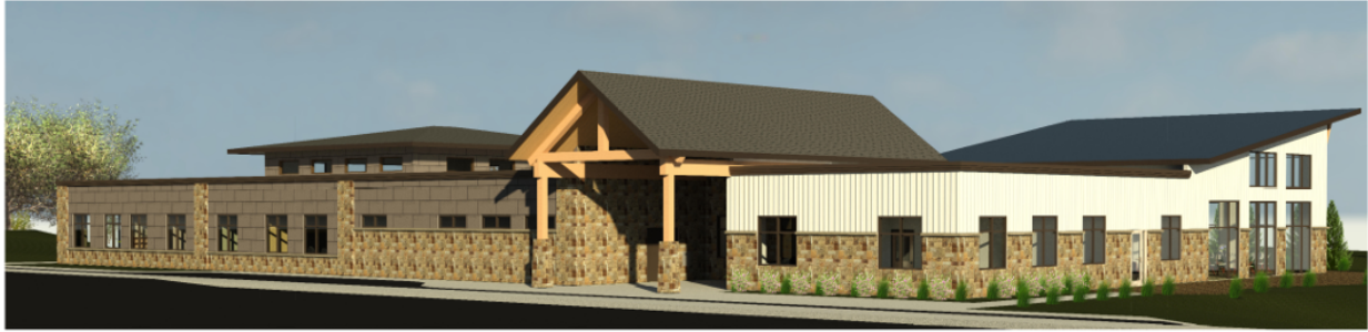
SOUTHEAST CORNER VIEW
